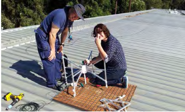
Final year Curtin Electrical and Computer Engineering student Mia Walker is assisted by ICRAR engineer Mr David Emrich in the roof-top installation of an interferometer designed for learning and outreach purposes.
